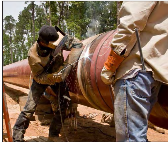
Cross-country pipe welding.
